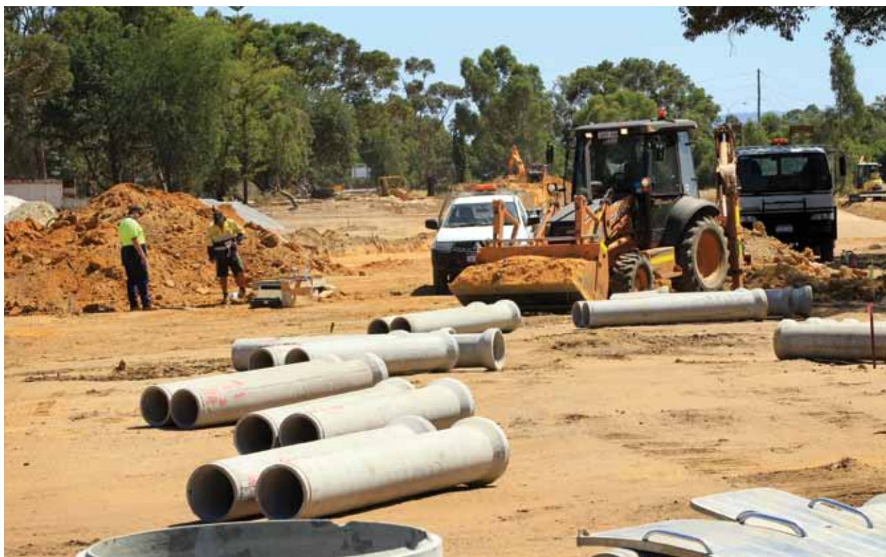
New Ranford Road works will provide access to Forrestdale Business Park
