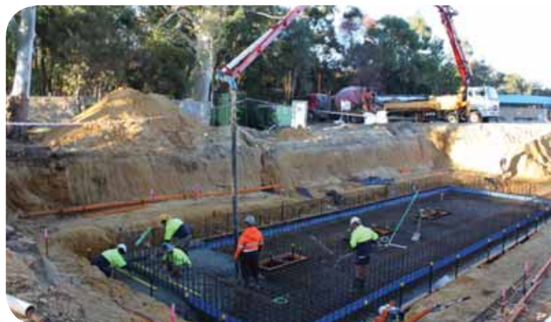
Armadale Aquatic Centre redevelopment underway
