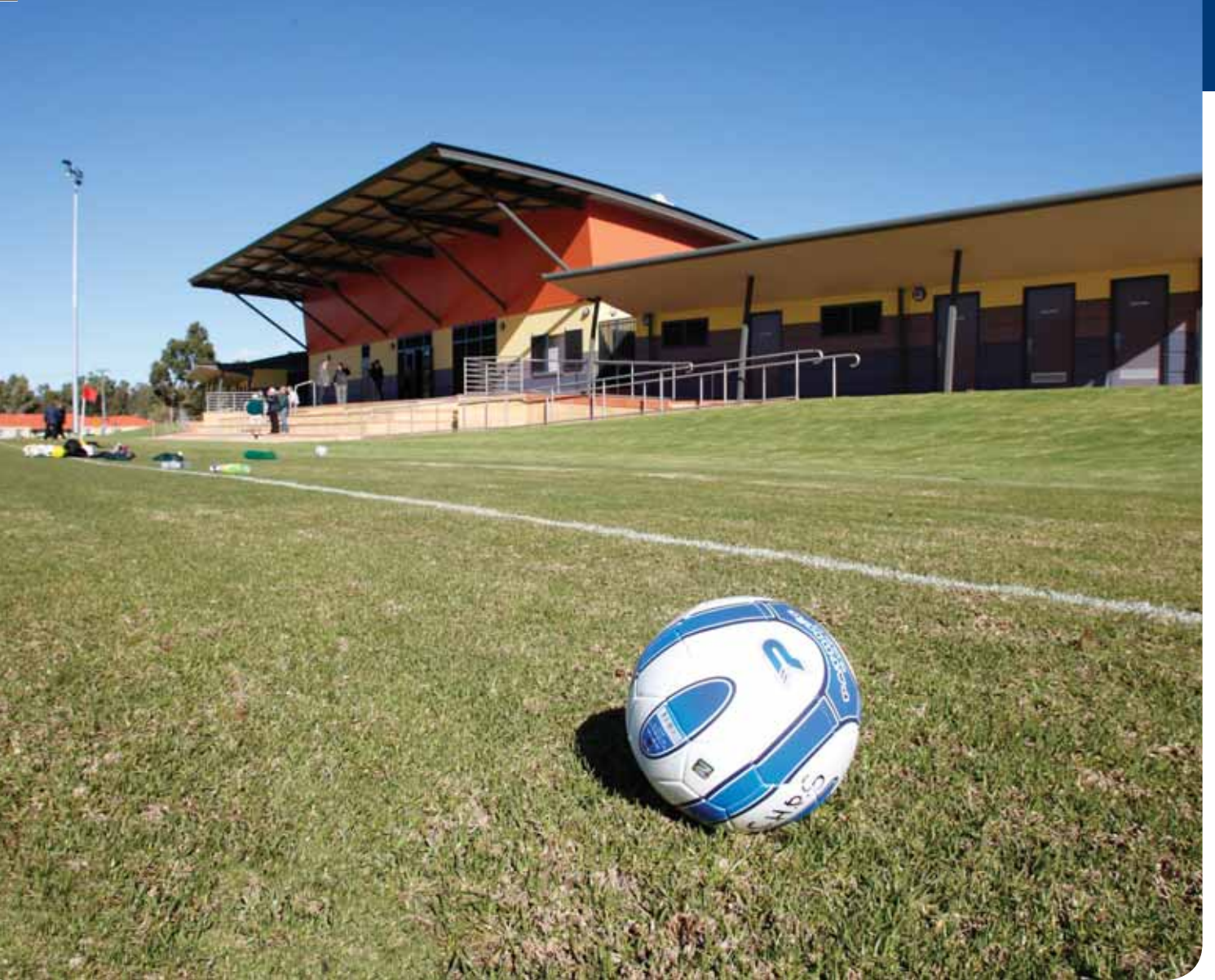
Frye Park playing surface includes a hi-tech irrigation system that automatically shuts down when it rains
