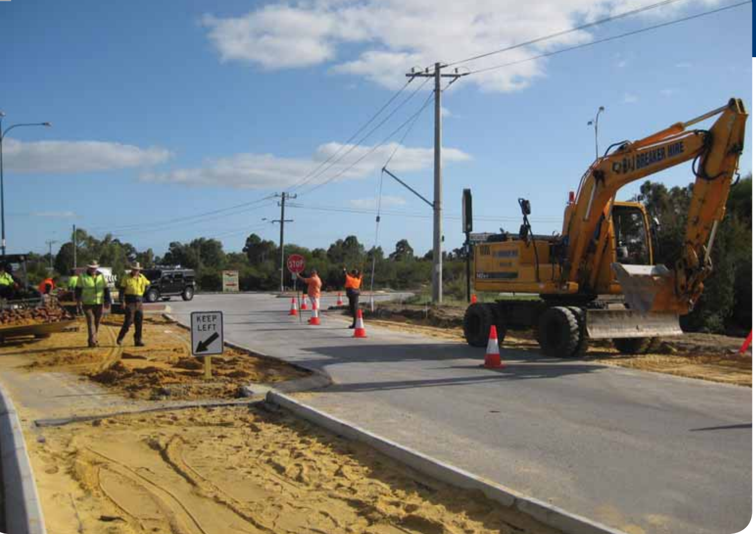
Warton Road gets upgraded
