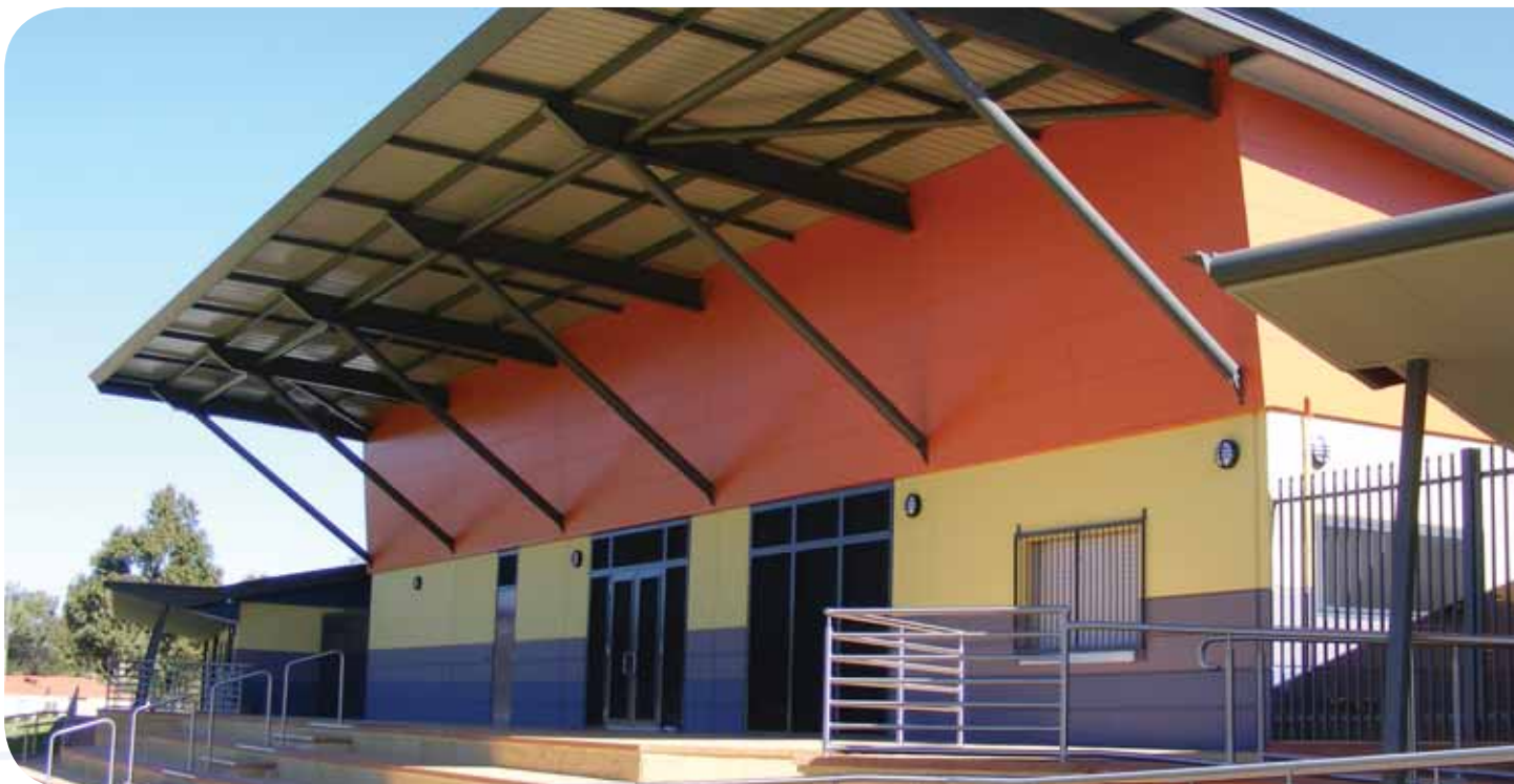
The Frye Park redevelopment is a state of the art community sports facility
