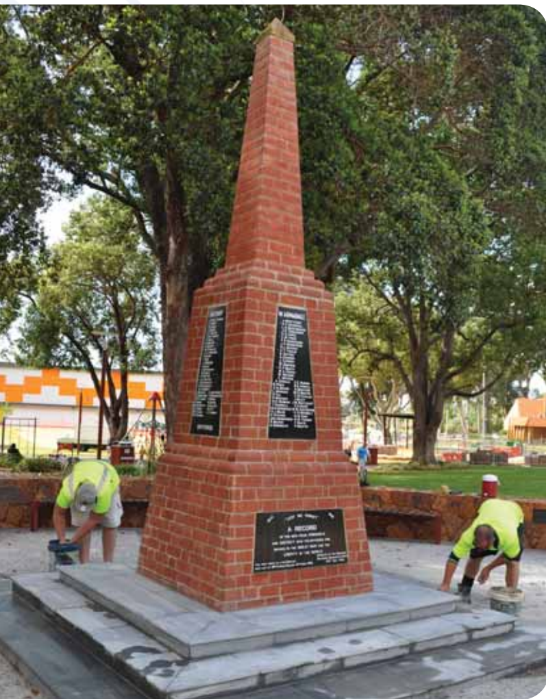
The upgrade works at Memorial Park include accessible pathways and seating.
