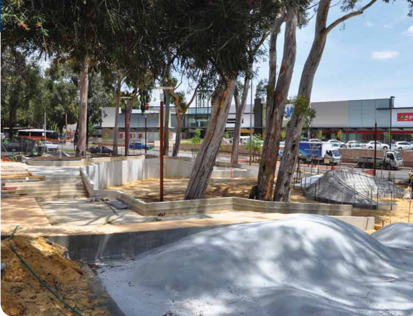
The Youth Activity Area is under construction
