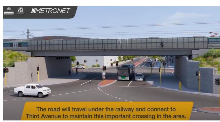
Figure 46 New Davis Avenue underpass (view from realigned Third Avenue) with new signalised intersection with Railway Parade (source: METRONET YouTube Channel - https://www.youtube.com/watch?v=dBTZAVGRKUs)
