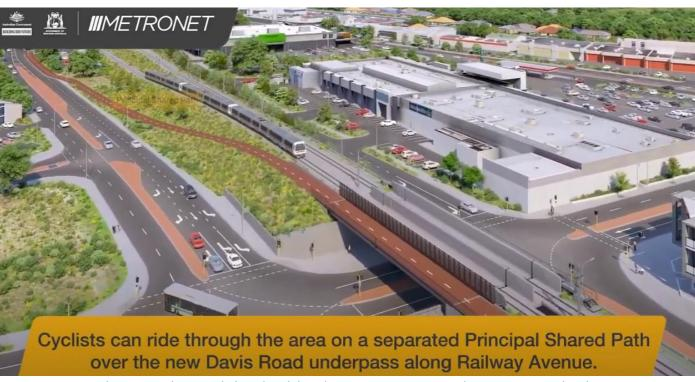
Figure 47 New grade-separated Principal Shared Path bicycle route connection over the new Davis Road underpass (source: METRONET YouTube Channel - https://www.youtube.com/watch?v=dBTZAVGRKUs)
