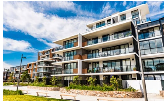
Image: Building height provisions in the Precinct SP will achieve specific interface outcomes where appropriate
