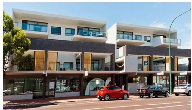
Image: Building height provisions in the Precinct SP will achieve specific interface outcomes where appropriate
