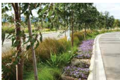
Bioretention swales provides water infiltration and ecological benefits
