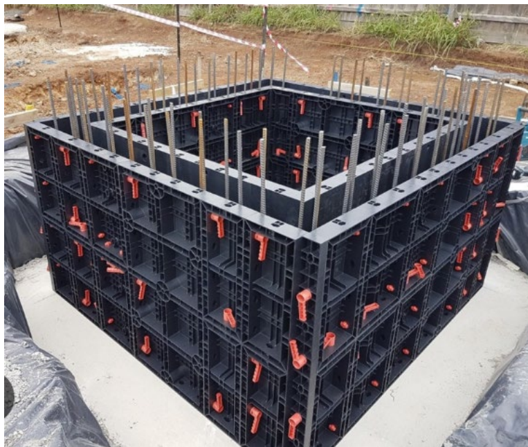
Figure 5: Example of Lift Core Formwork Systems
