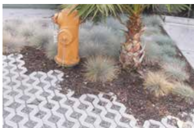
Permeable paving around vegetation and tree planting
