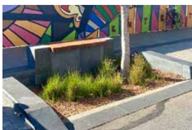
Small rain garden filters and treats storm-water run off
